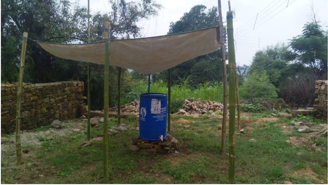
Illustration II: Simple portable rainwater harvesting system
