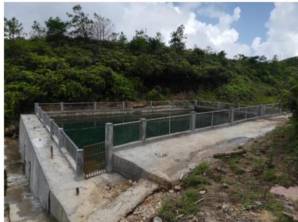
During Work Picture
