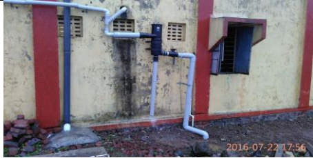
Recharge structure at orphanage
