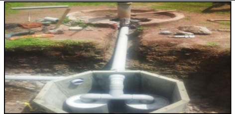
Filtration and recharge pit
