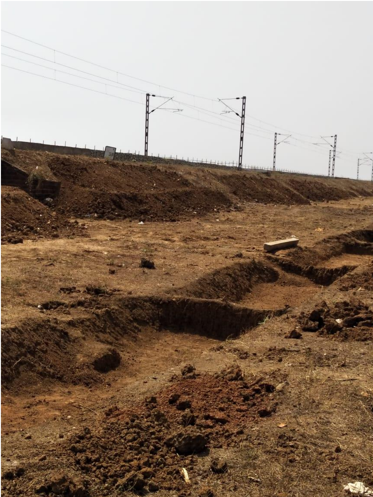
Pic. 27 – View of finished site
