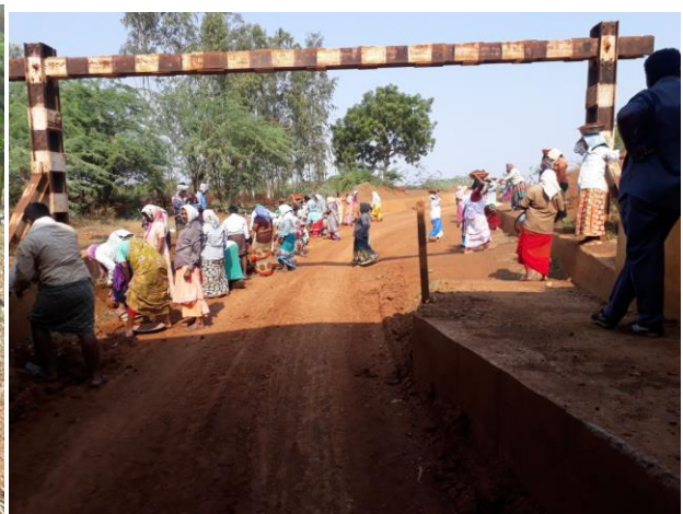
Pic. 14 – Desilting of bridge under progress
