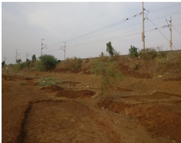
Pic. 15 – Cess repair under progress
