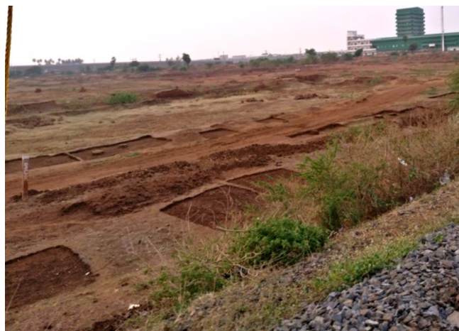
Pic. 16 – Digging of soil to repair cess
