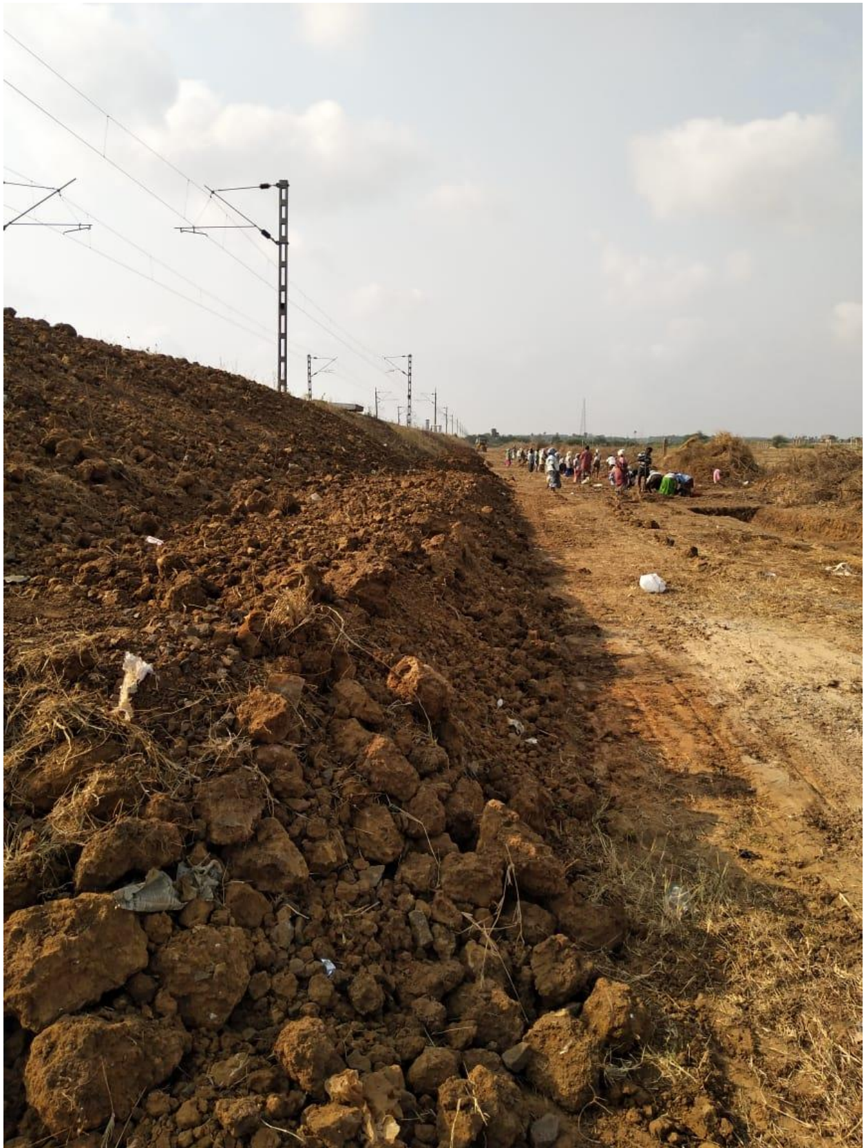
Pic. 30 – Another view of work under progress
