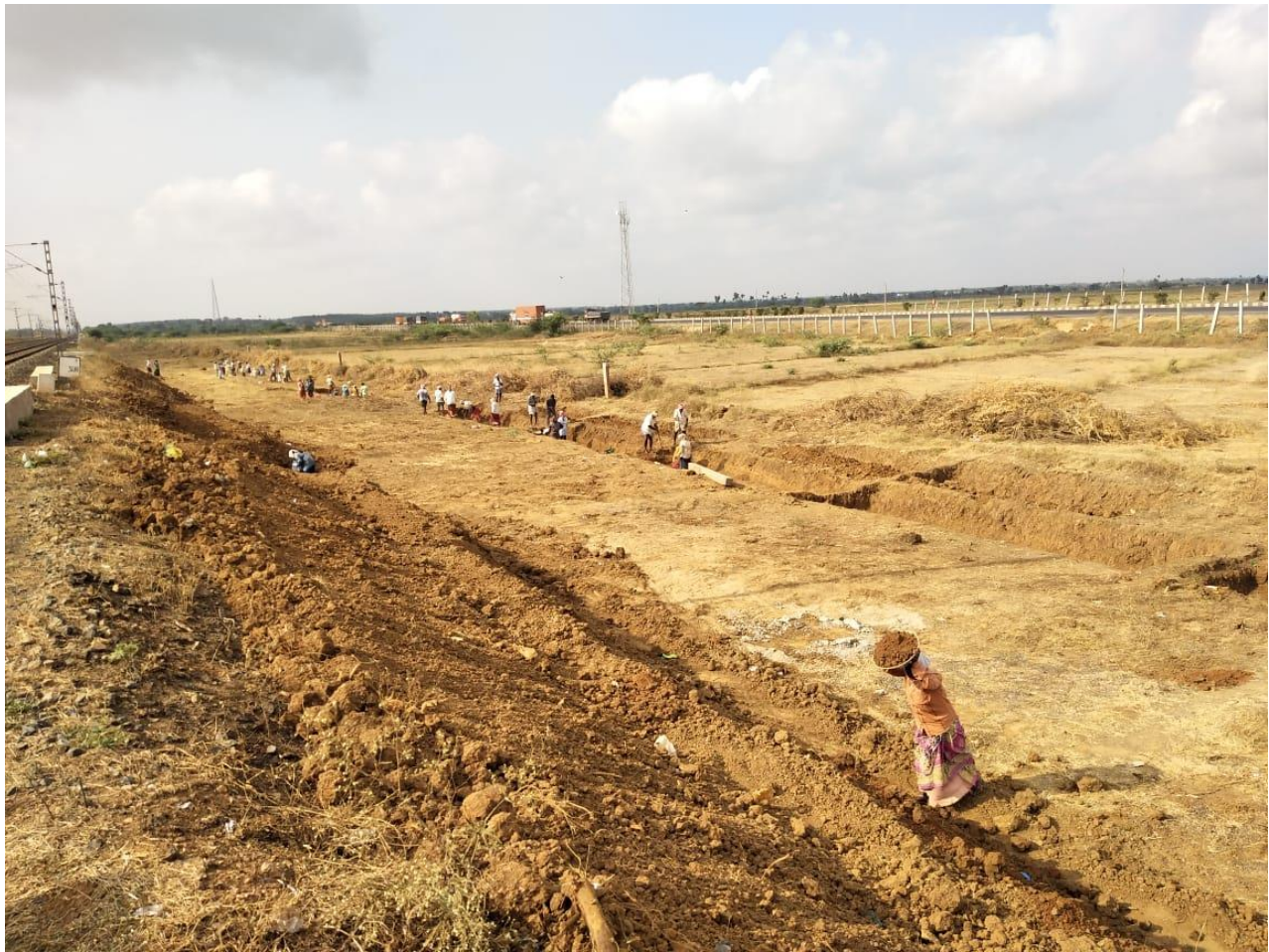
Pic. 29 – View of work under progress
