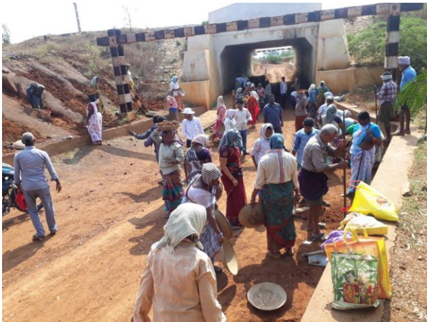
Pic. 13 – Labour clearing silt
