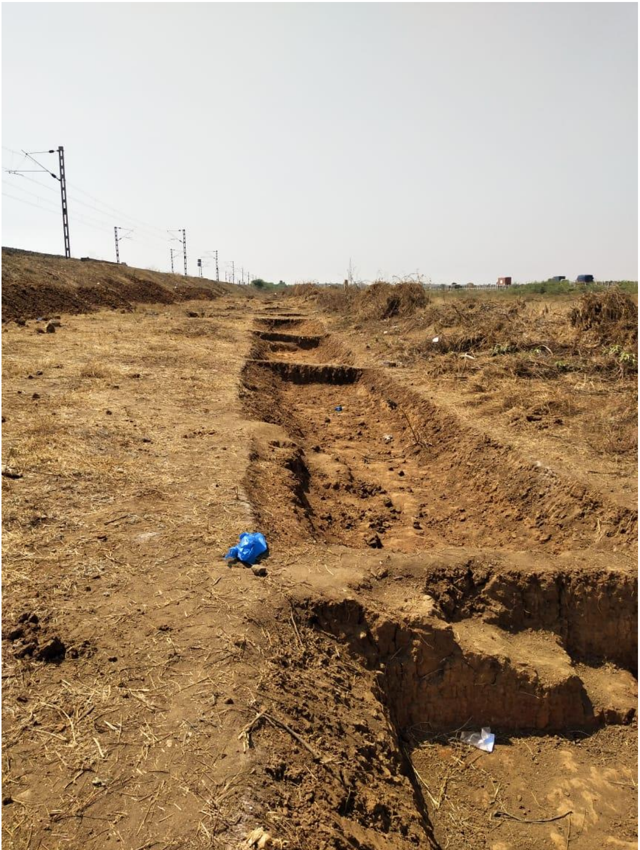
Pic. 28 – Another view of finished site
