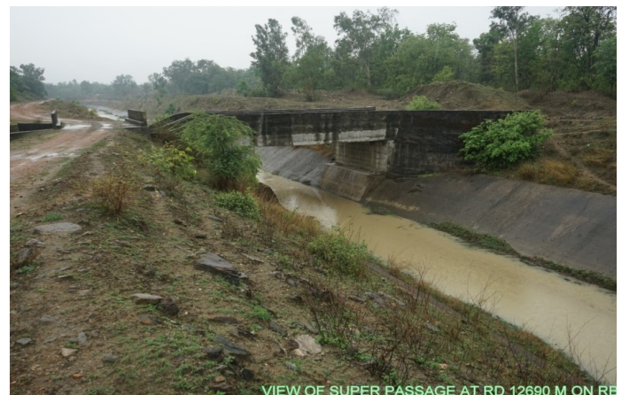
VIEW OF SUPER PASSAGE AT RD 12690 M ON RE
