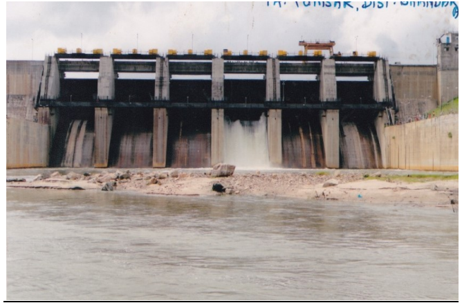
Earthen Dam across River Bawanthadi, Live Storage- 217MCM
